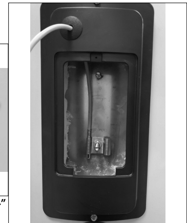
Figure 22 - Sensor Clip on the Lower Stud
